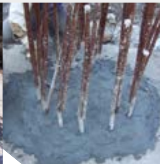
Installing a fillet and smoothing the area with KÖSTER R4 Mortar.
