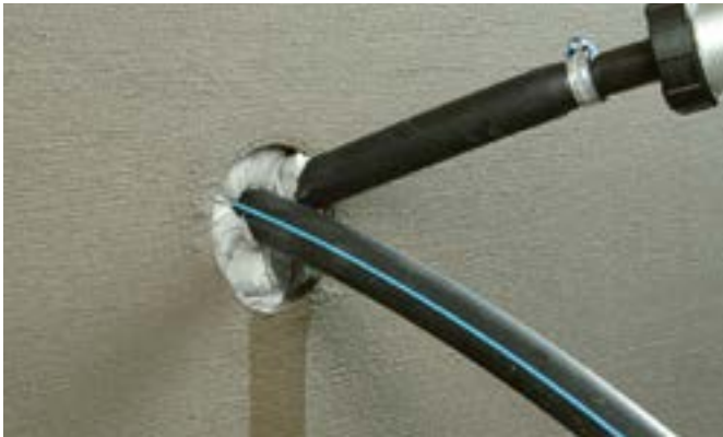
KÖSTER KB-Flex 200 is installed into the void using the KÖSTER Special Caulking Gun.
