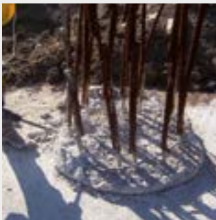
Removing protrusions, cleaning the pile head.
