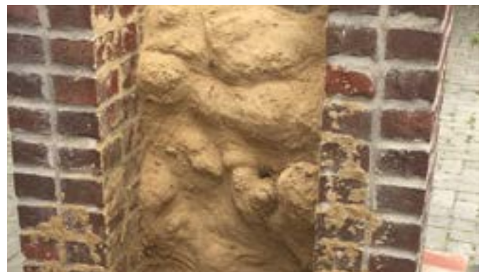
Curtain Injection (rear view)
