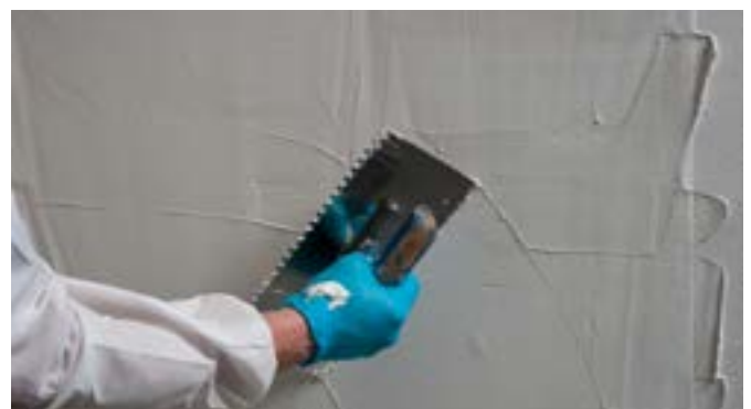
First layer of KÖSTER 21 with KÖSTER Flex Fabric
