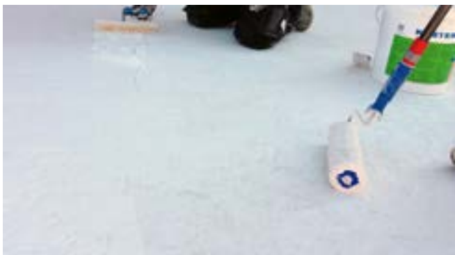
Application of the second layer of KÖSTER 21
