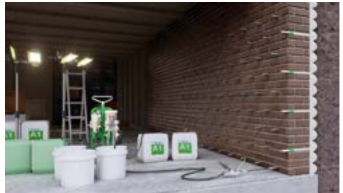
Curtain Injection of Masonry
