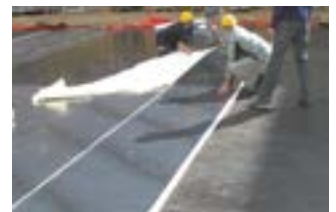
Waterproofing with KÖSTER KSK
