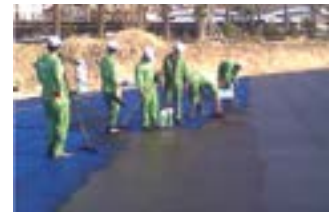
Waterproofing with KÖSTER Deuxan 2C
