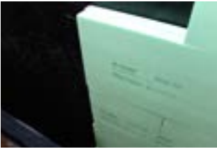
Insulation boards can be easily attached with two-component KÖSTER PMBCs. It is important that the insulation boards are fully bonded.
