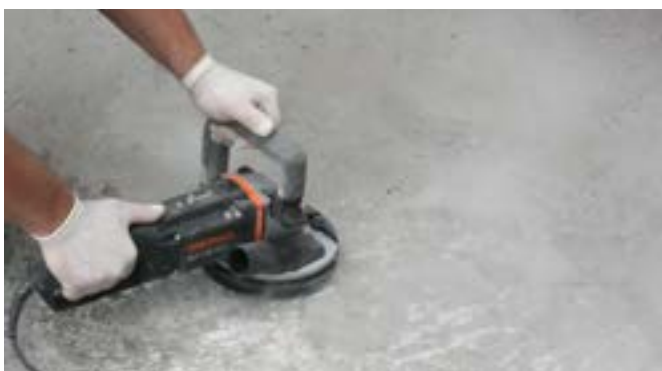
Substrate preparation
